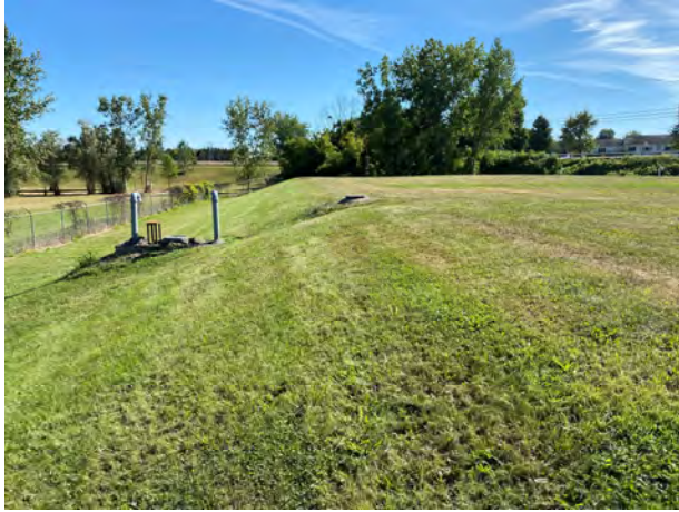
South Byron Filter Beds and Aeration Structure
