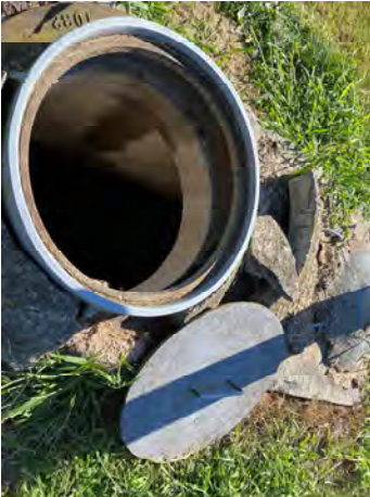
South Byron Aeration Structure MH
